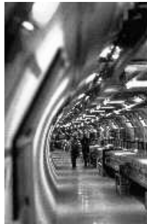
Inside the LEP Tunnel
